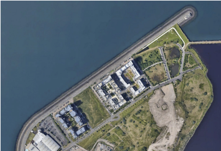
Aerial image of Western Harbour waterfront properties. (Google Earth, 2022)
