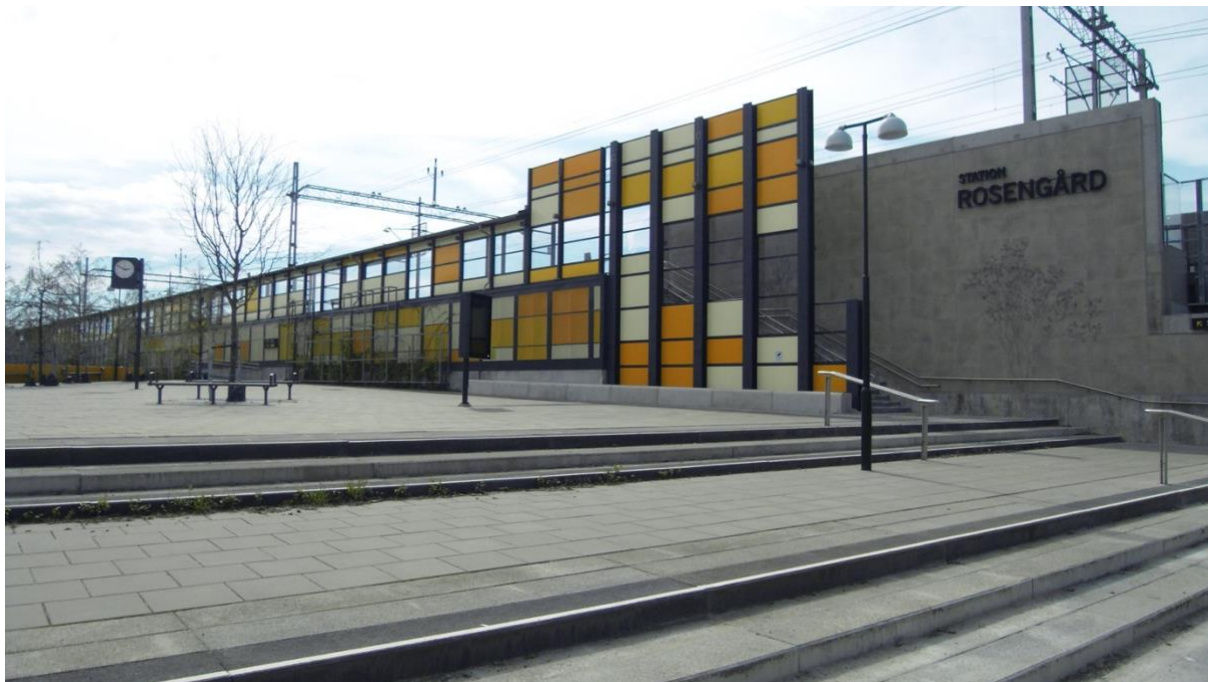
Figure 2. Rosengård station. Source: Jin Zan (Wikimedia Commons)
